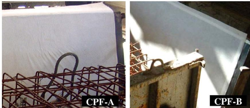
Fig. 2. Application of filter-drain A (CPF-A) and filter-drain B (CPF-B) on box-culverts outer side walls A and B.
