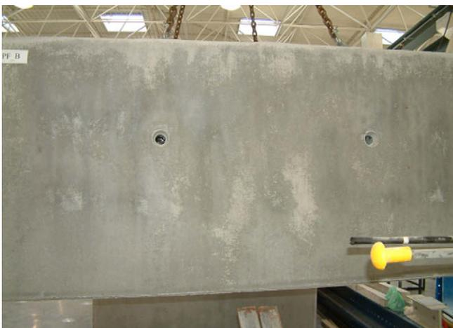
Fig. 6. Concrete surfaces resulting from application of CPF-B on CC box-culvert.
